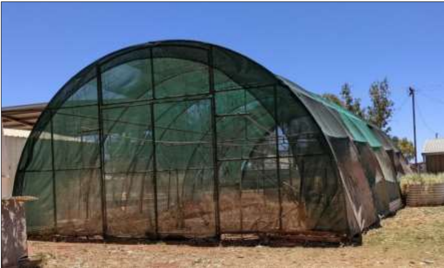
Figure 2.5: Out-of-commission greenhouse at Burringurrah Remote Community School, 31 October 2022
